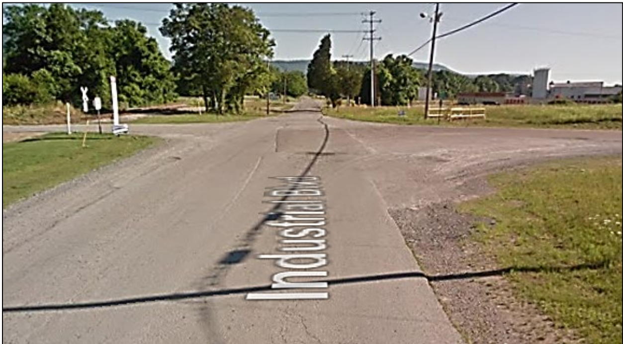
BEFORE – Image of intersection of Industrial Blvd. & Godsey Drive (Google - June 2018)
