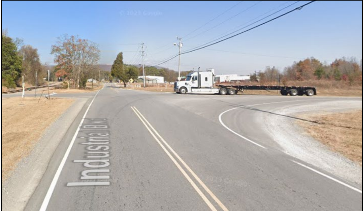
AFTER - Image of intersection of Industrial Blvd. & Godsey Drive (Google – August 2023)
