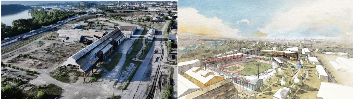
(Left) U.S. Pipe/Wheland Foundry site as it is today and (Right) a rendering of what is to be the new stadium
